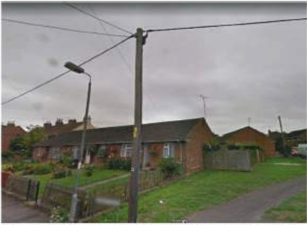
240v LV pole; note the yellow "Danger of Death" sticker and the grey plastic tube on the side, indicating underground cabling.
