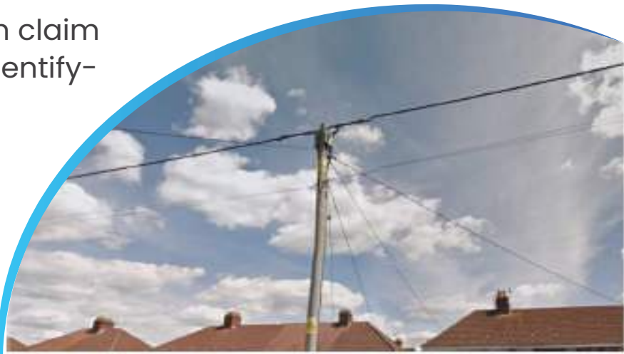
LV electricity pole with both electricity wires and telegraph wires coming off it. The electricity wire is at the very top of the pole and the thinner telegraph wires are located lower down on the pole. They also spread out from the pole whereas the electricity wire forms a straight line.
