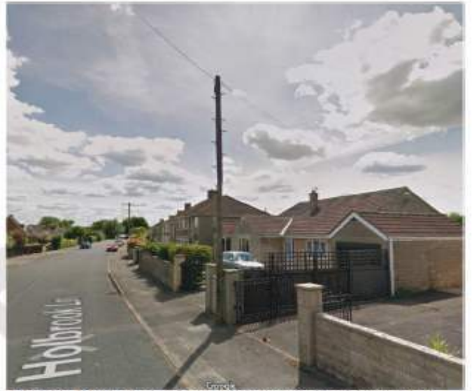
Telegraph pole; note no "Danger of death" sticker and small metal rungs towards top. Cables are thinner than electricity cables.
