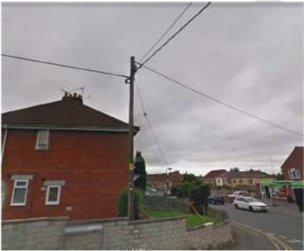
240v LV pole; note the yellow "Danger of Death" sticker and the grey plastic tube on the side, indicating underground cabling.
